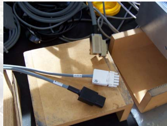
Connections to turbo, dc power out and ac power in
